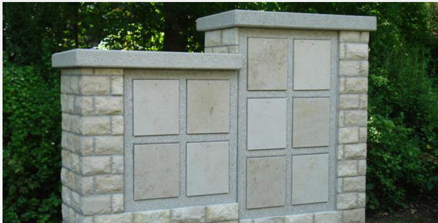
Urnenwand / Kolumbarium in Steinmauer
